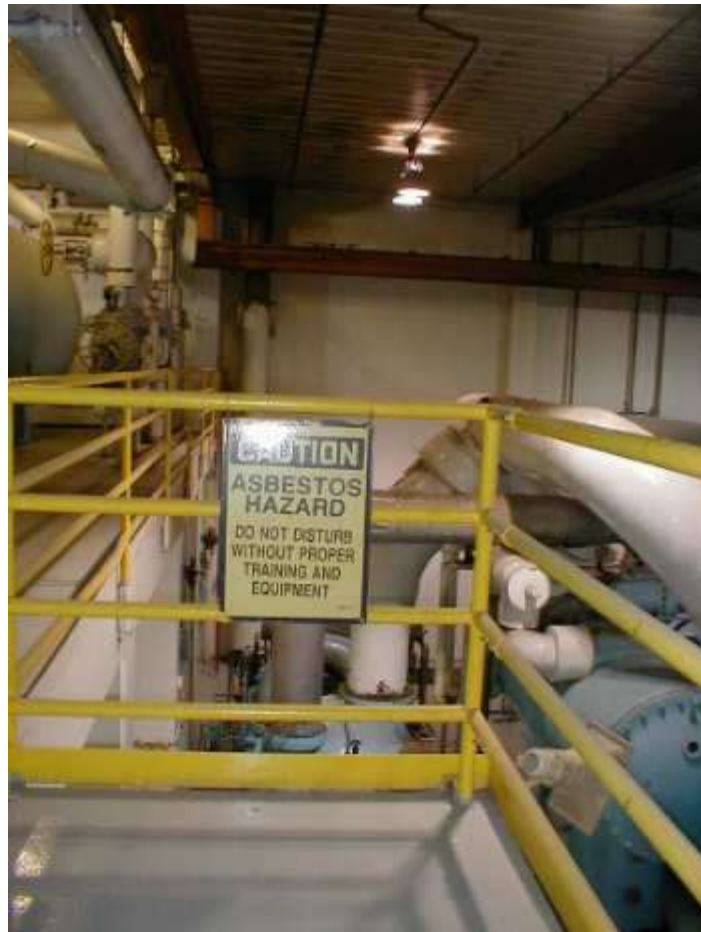
These are pictures of the interior of the facility.
